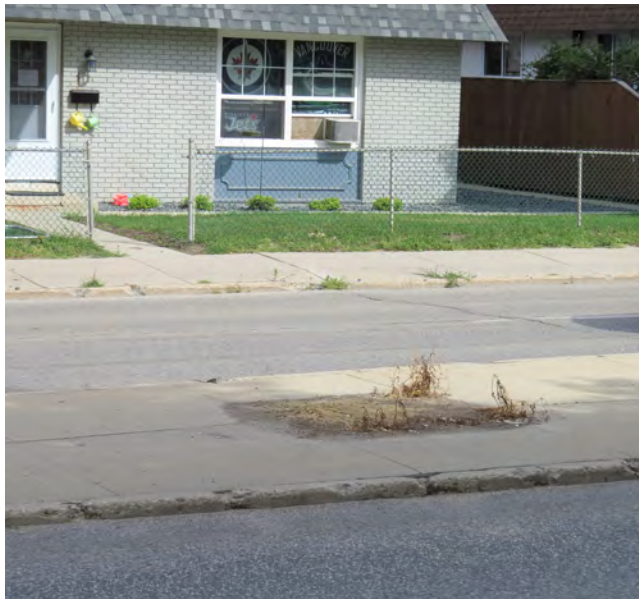
Figure 27: An example of a vacant planting sites in Winnipeg.
